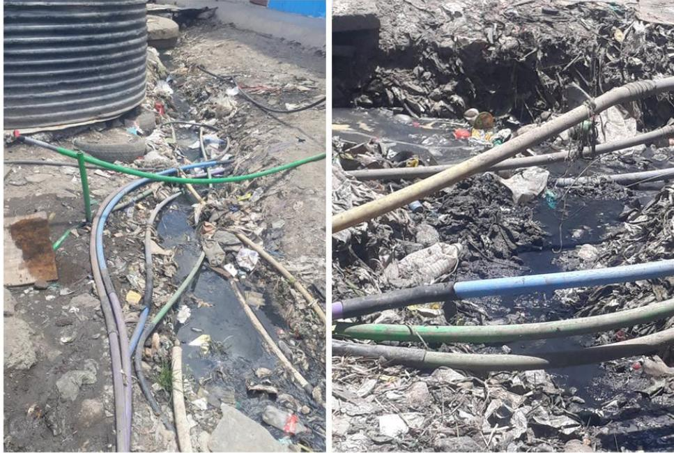
**Figure 4.1: Clean water pipes laid in open sewage and highly polluted environment in Kibera informal settlements**
